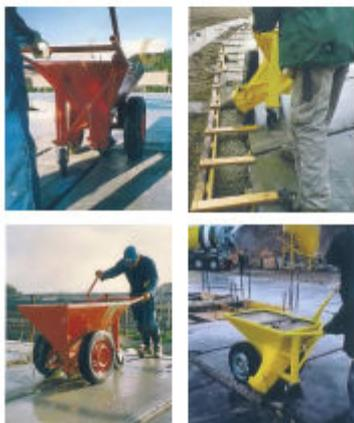
For pouring of strip foundation/channel hollow core slab floors.
